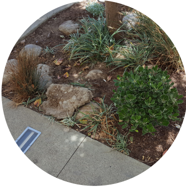
Planted Storm Water Drainage
